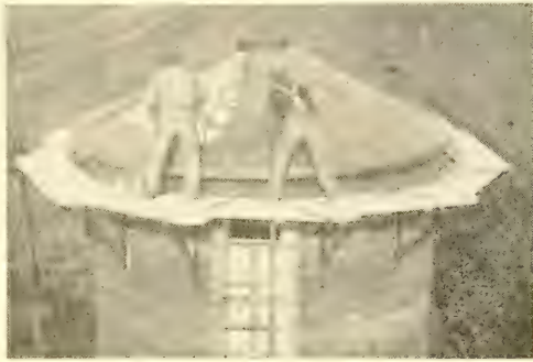
Completing a Conical Roof
